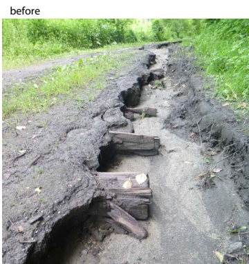
The Cross Vermont Trail located on the Montpelier & Wells River railbed where the town owns the old bed in Marshfield was heavily impacted - exposing the rail ties! The town has completed a major rebuild this Fall. Next year CVTA will work with the town to complete further improvements at the trailhead here, and also to upgrade additional sections of the railbed elsewhere.
