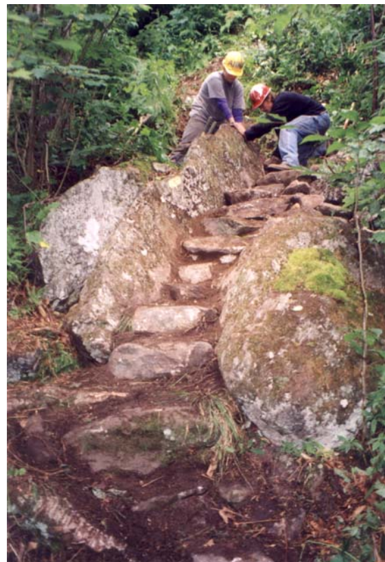
Trail Step Construction Credit: Luke O'Brien
